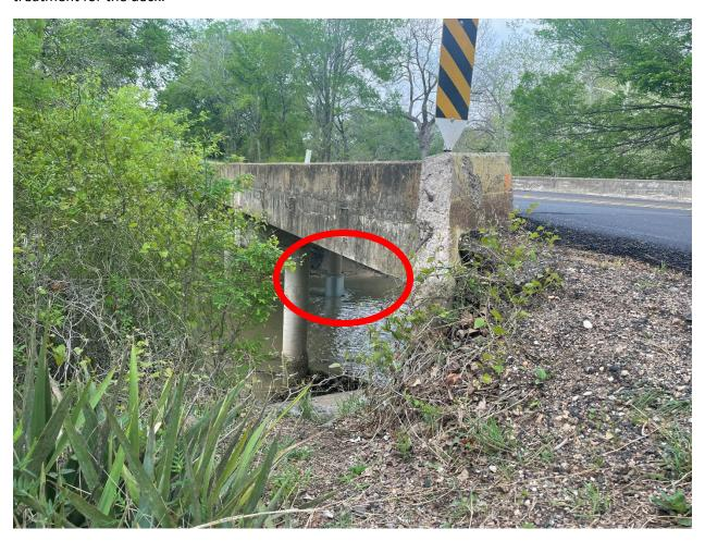
This dynamic along with the 2-foot drop in the creek bed has the potential to undermine the bridge. Since the expanded scope of work now requires entering the water of Nolan Creek to rehabilitate the bridge, the scope of the environmental review now has an additional requirement for a TPWD mussel survey.
