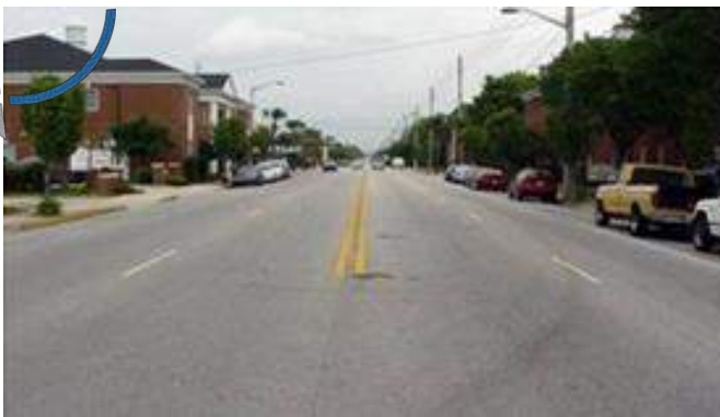
Figure 3-3: Road Diet Implemented on a 4-Lane Street
