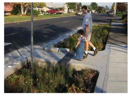
Green and complete streets manage a street's stormwater runoff by using green infrastructure, and provide safe and accessible routes for all users.
